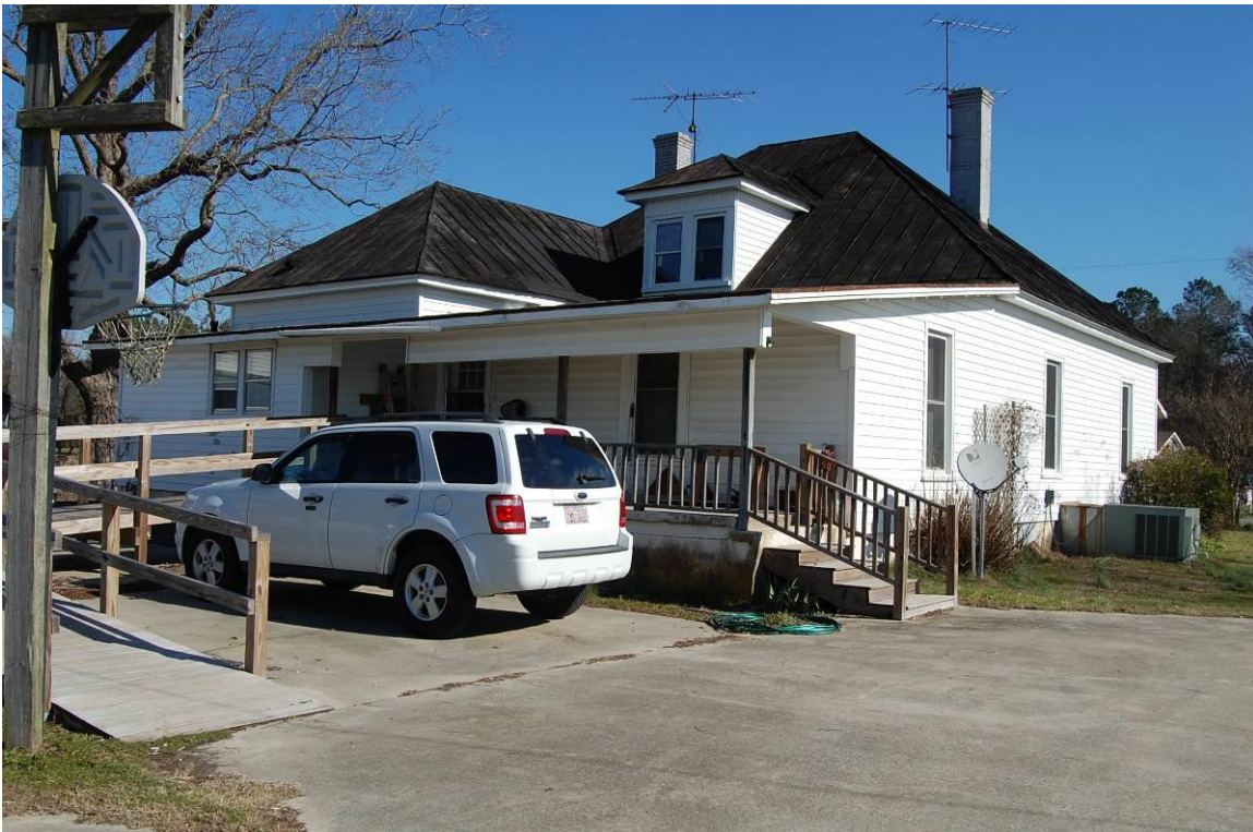
Figure 124. West rear and south side elevations of house
