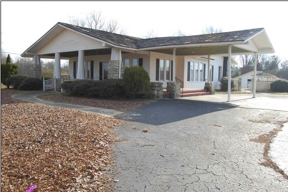
Figure 156. North front and west side elevations of house
