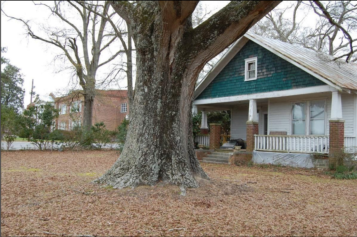
Figure 18. Looking west at southwest front elevation of teacherage, at right, and Contentnea School, at left
