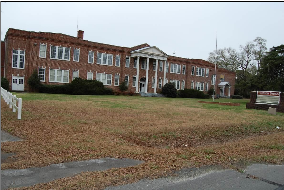
Figure 15. Southwest front elevation of original central block of Contentnea School
