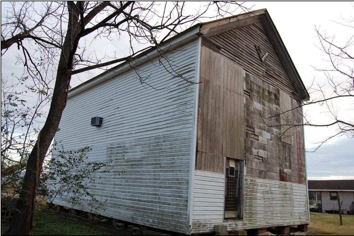
Figure 185. Northwest rear and northeast side elevations
