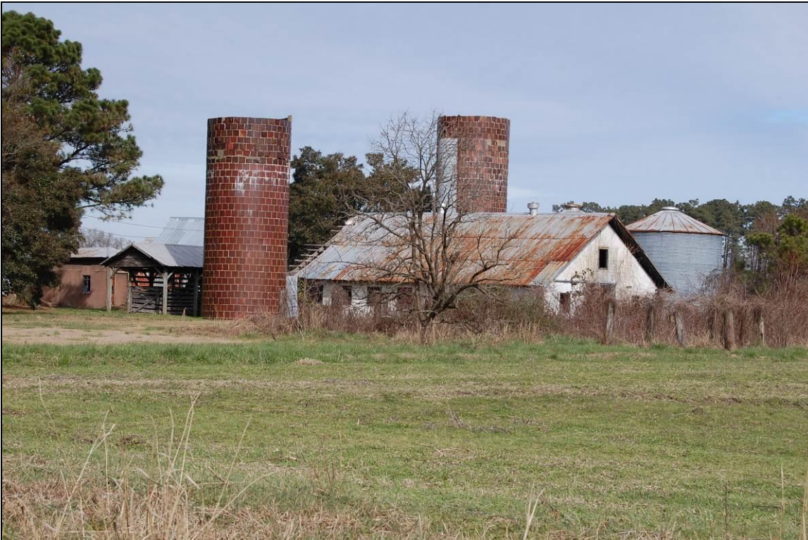
Figure 8. Looking northeast from south of house at small open shed at left, dairy barn at center, and silos at center and right
