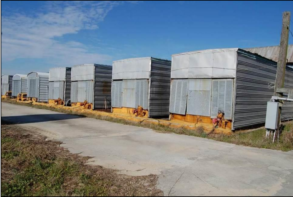
Figure 131. Looking northwest at south flank of bulk barns
