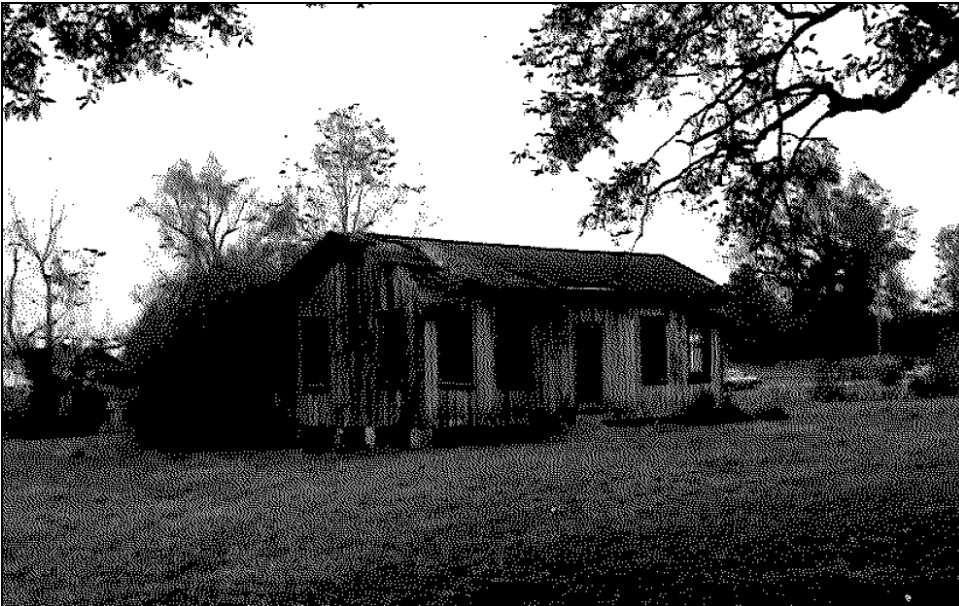
Figure 194. Graingers Railroad Section House, looking northwest in 1993 (photographer: Robbie Jones)
