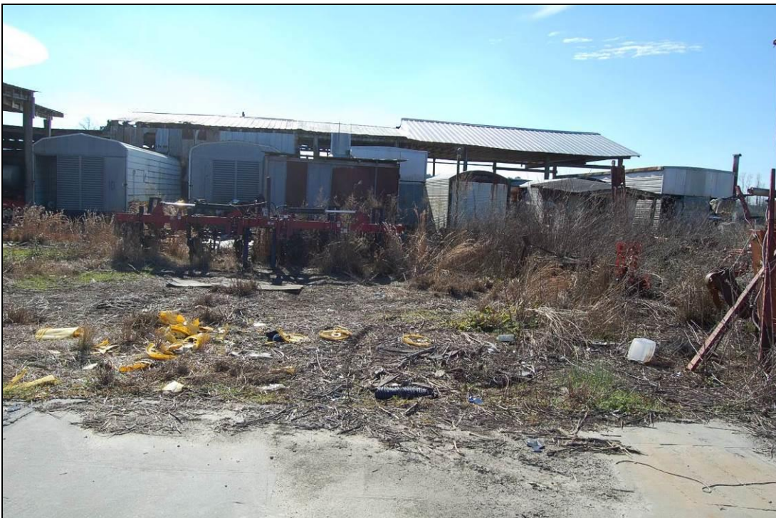
Figure 134. Looking south at central shed and bulk barns lining its north side
