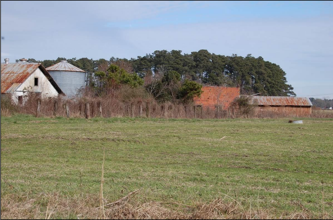
Figure 9. Looking east from south of house at dairy barn and silo at left, clay-tiled walls of roofless tobacco barn at center, and shed at far right
