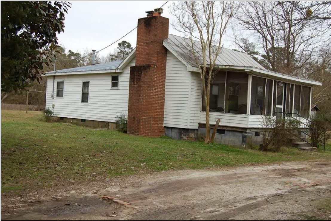
Figure 88. Eliza Dawson Farm, west side and south front elevations of house
