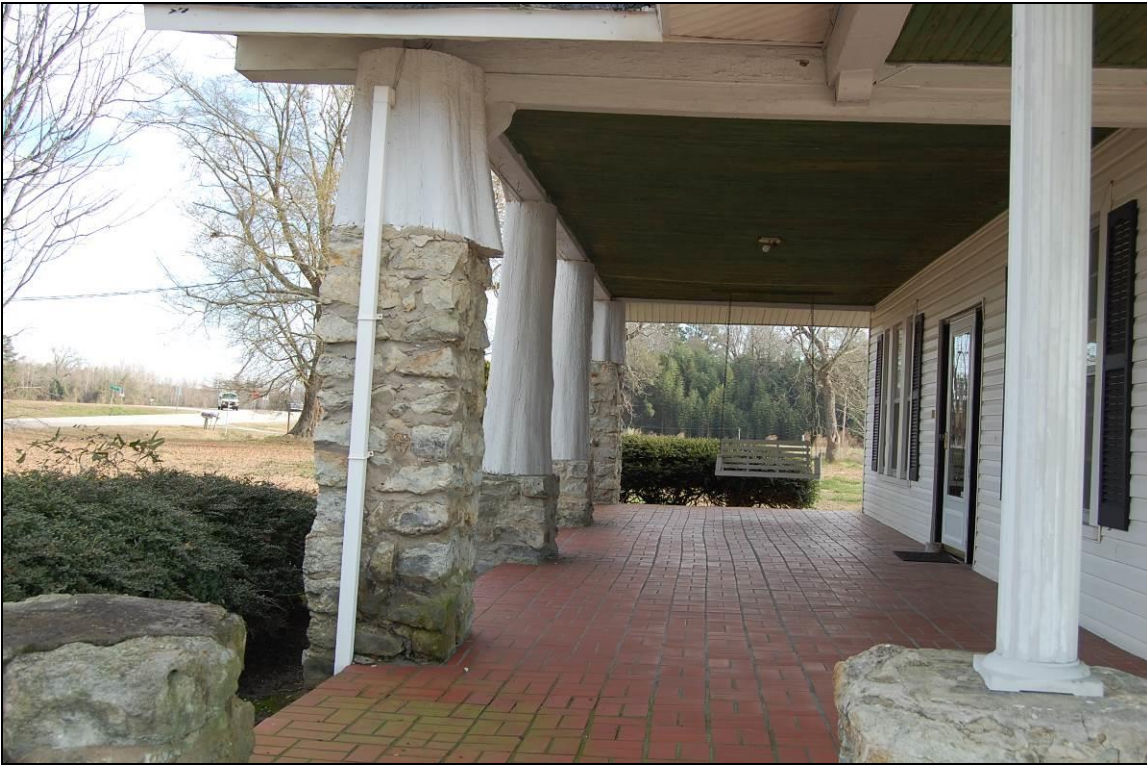
Figure 157. Looking east at front elevation and porch of house
