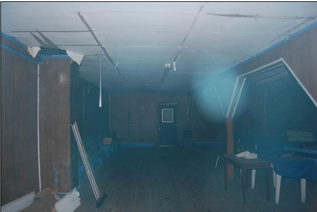
Figure 190. View through rear door window into downstairs room
