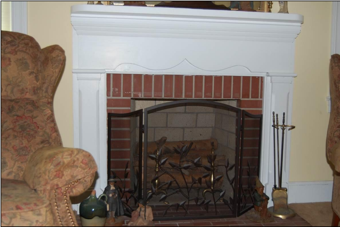
Figure 142. Post-and-lintel mantel shifted from front block of house to rear addition
