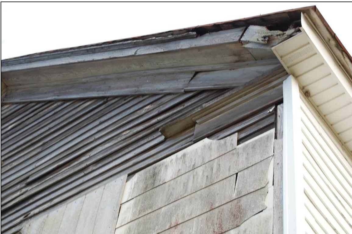
Figure 188. Northwest rear elevation cornice and cornice return
