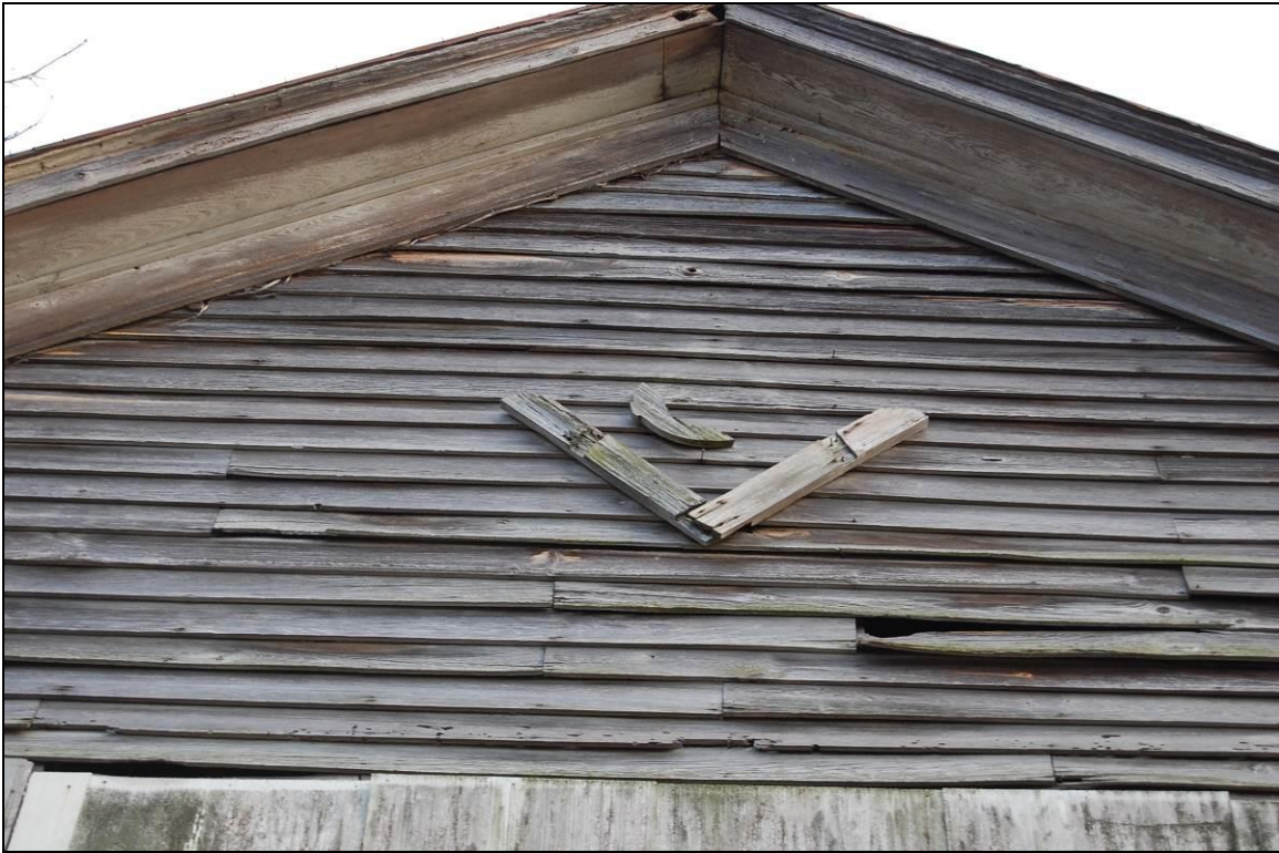
Figure 187. Northwest rear elevation weatherboards, cornice, and remnant of square-and-compass Masonic symbol
