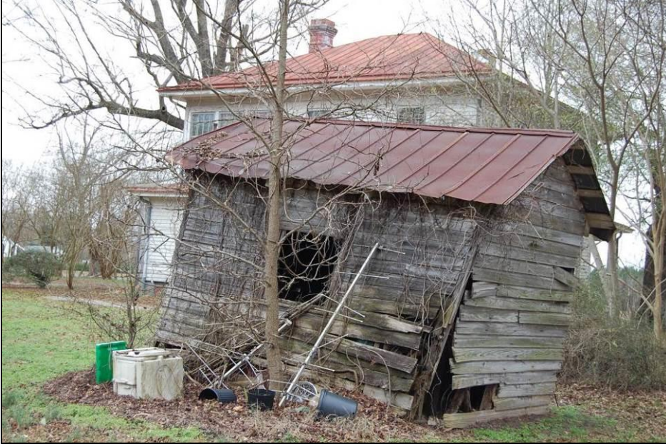
Figure 39. Toolshed, southeast rear and northeast side elevation
