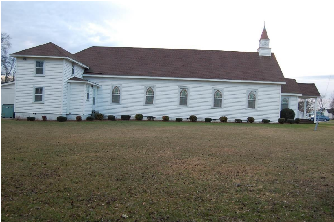
Figure 178. East side elevation of sanctuary with hip-roofed Sunday school wing at left
