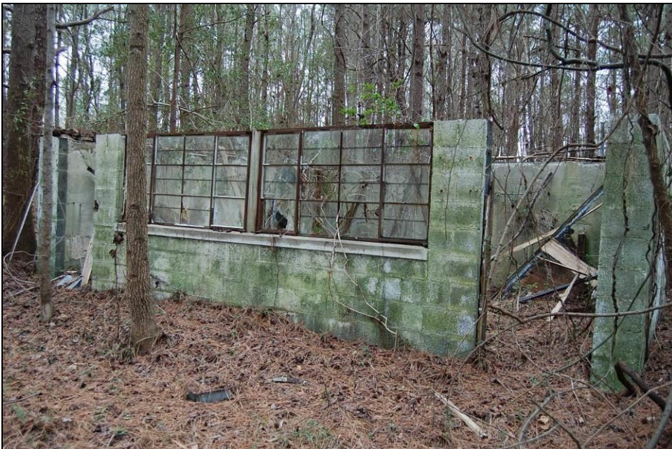
Figure 114. East-facing front elevation of concession stand
