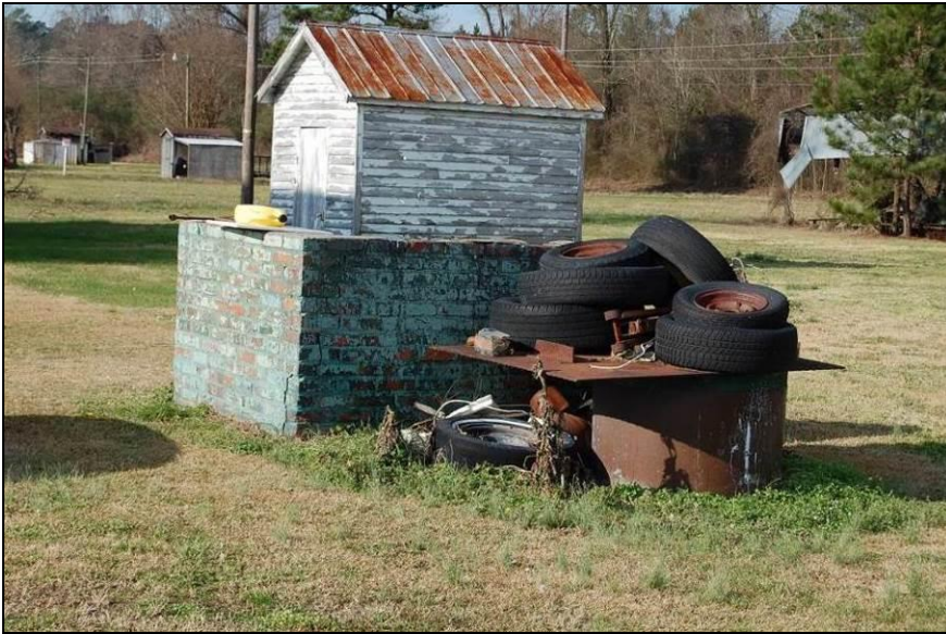
Figure 170. Looking northwest at covered shaft of well and walls of pumphouse
