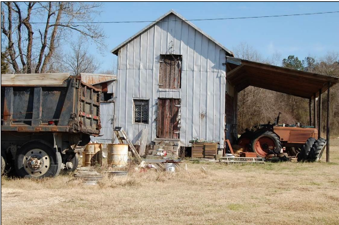
Figure 119. Looking east at packhouse at eastern edge of tract
