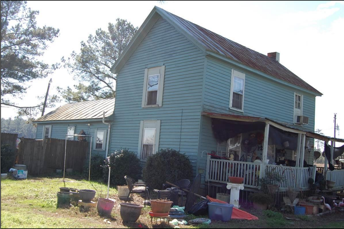
Figure 137. Northwest front and northeast side elevations of house
