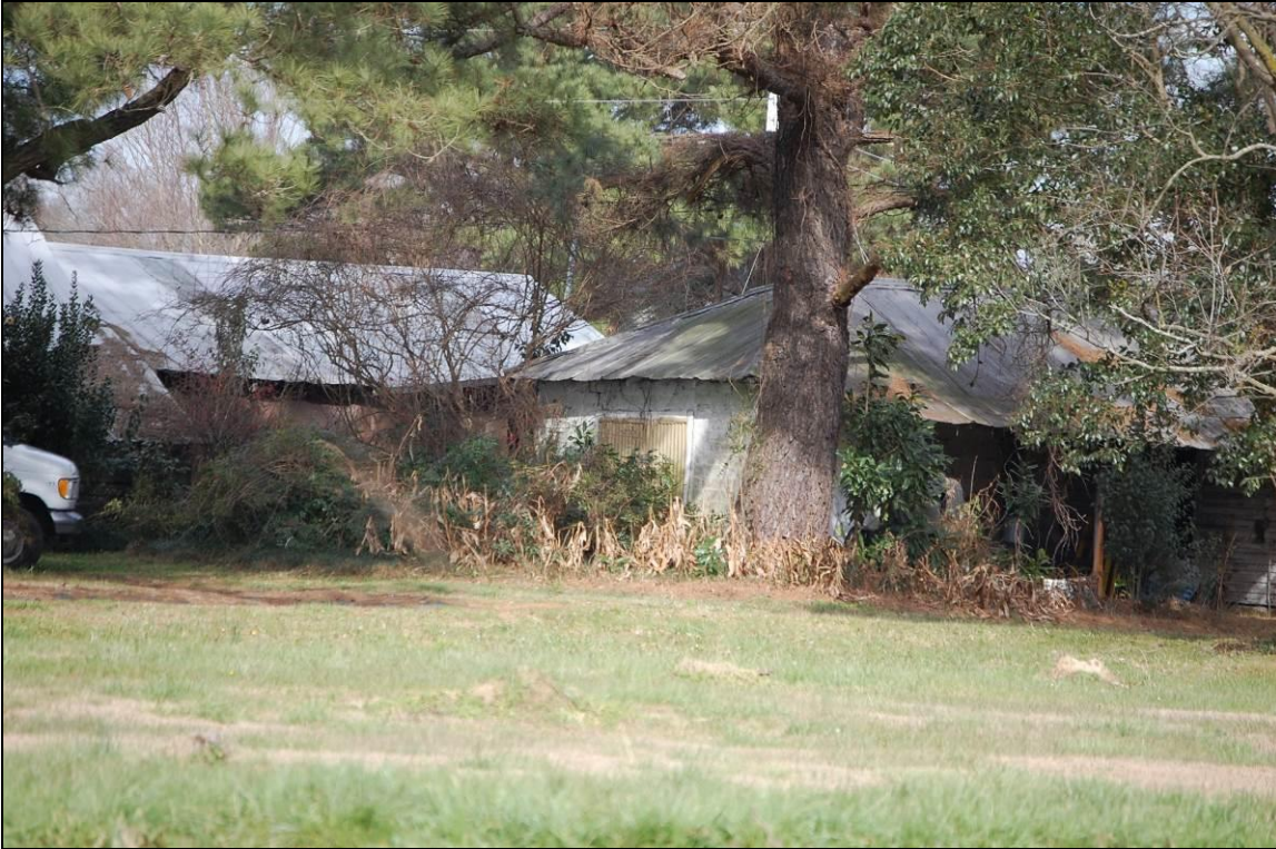
Figure 7. Looking northeast from south of house at concrete-block milkhouse
