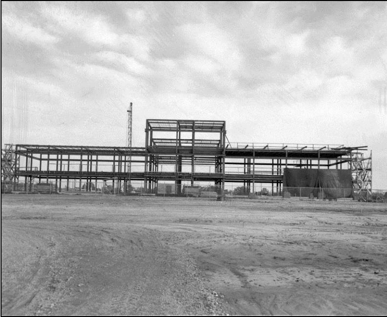
Figure 42. Plant at beginning of construction, 1951 (source: https://digital.lib.ecu.edu/1998 )
