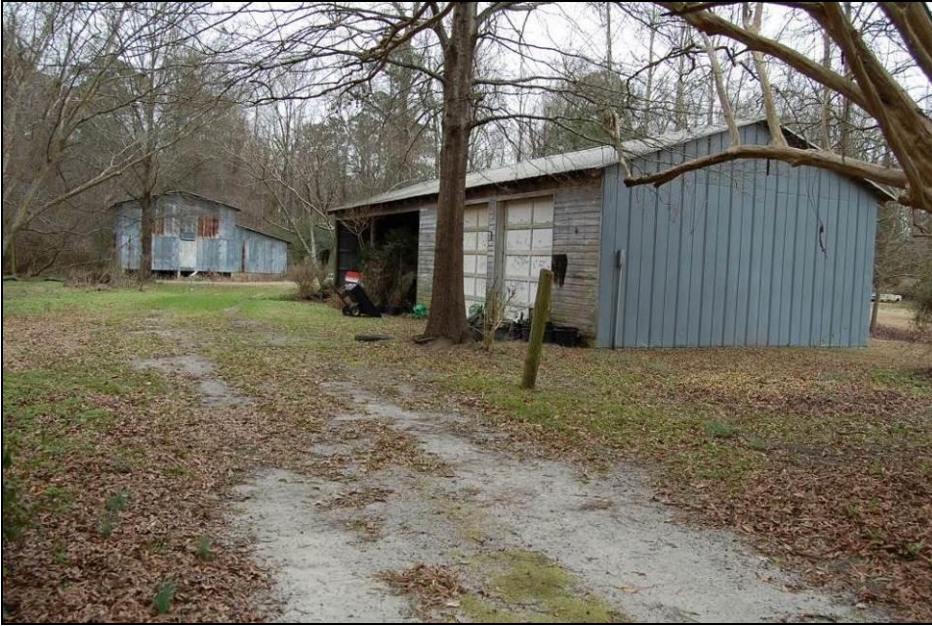
Figure 28. Shop/shed, northwest side and northeast front elevations; packhouse/barn in distance
