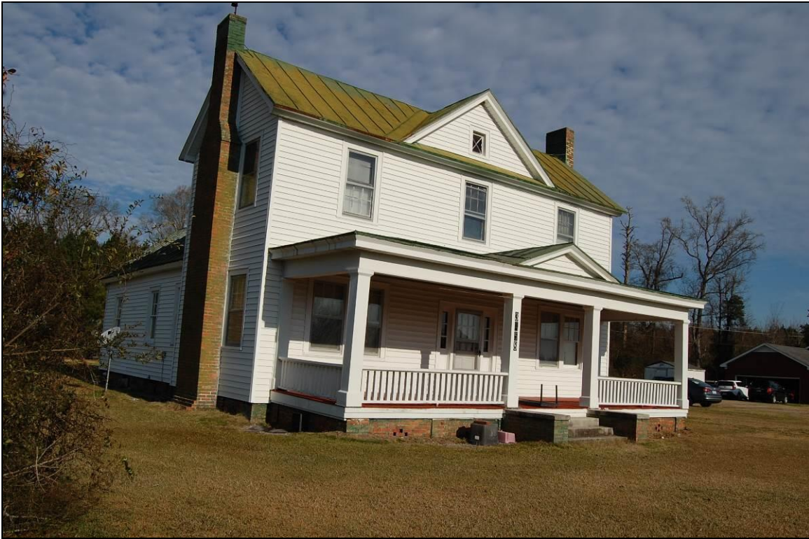
Figure 166. South front and west side elevations of house
