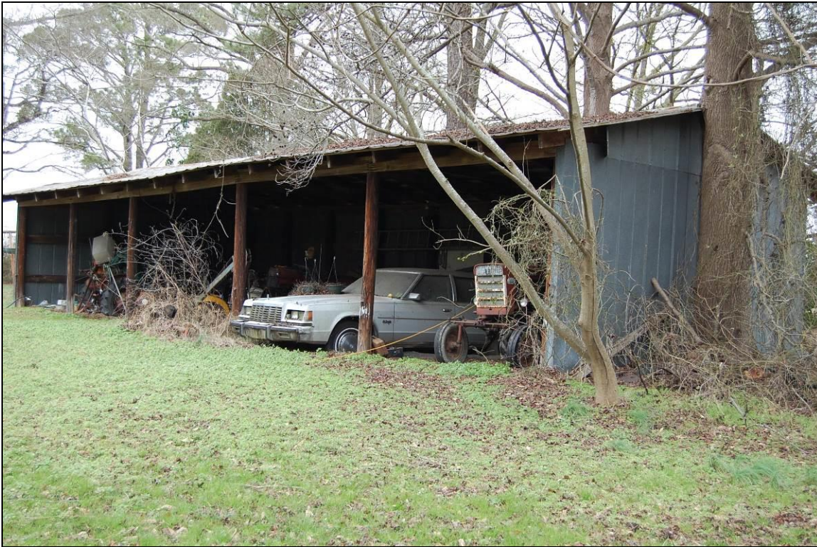
Figure 38. Farm equipment shed, southwest front and southeast side elevations
