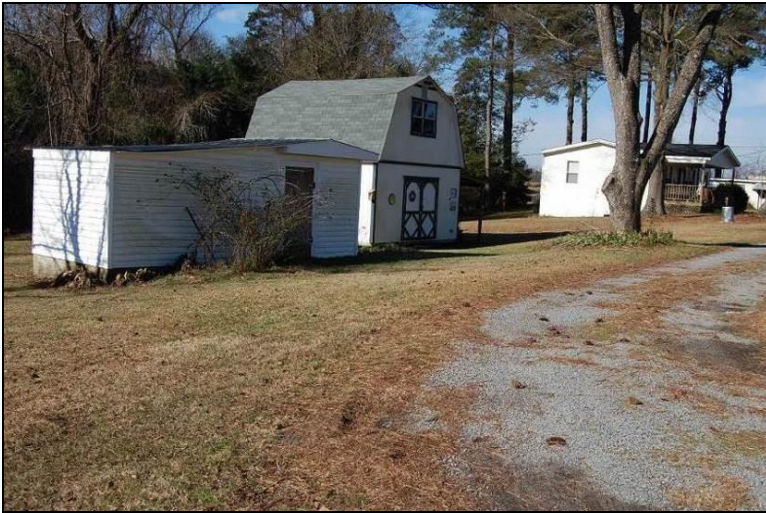
Figure 152. Looking southeast at pumphouse at left, manufactured shed at center, and manufactured house at right
