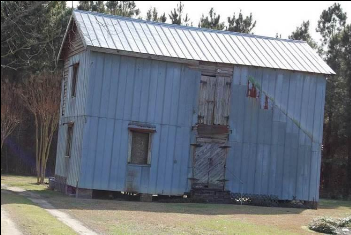
Figure 72. Willie Humphrey Farm, gable-end west and long north elevations
