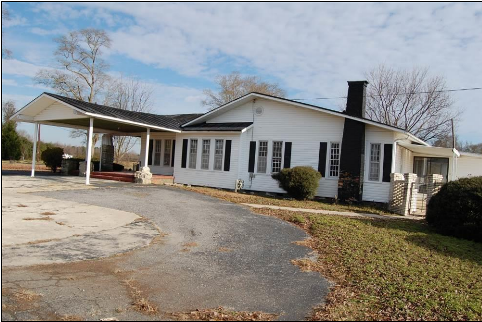
Figure 159. West side and south rear elevations of house
