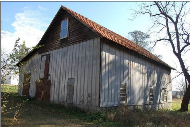
Figure 151. Looking northeast at packhouse
