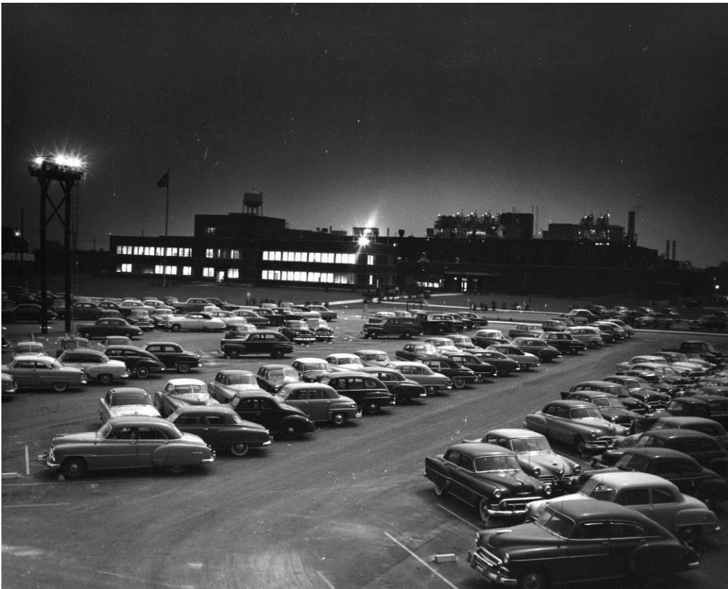
Figure 55. Looking northeast at office building and front of plant, early/mid-1950s (source: Hagley Museum and Library at http://cdm16038.contentdm.oclc.org/cdm/singleitem/collection/p16038coll2/id/1300/rec/1 )
