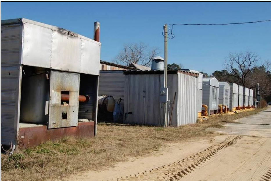
Figure 132. Looking northeast at southern row of bulk barns
