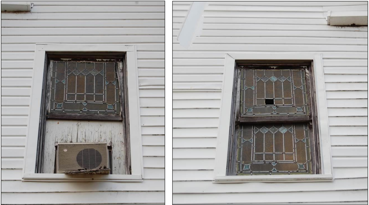
Figure 183. Southeast front elevation windows
