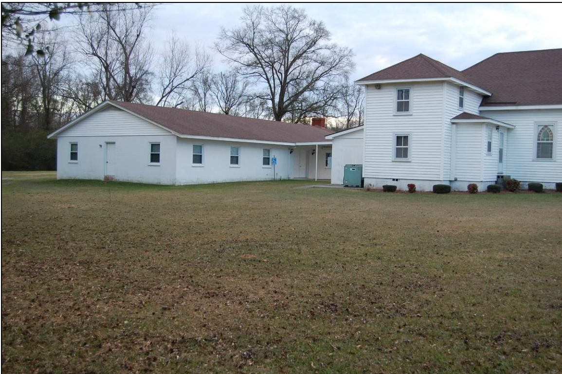
Figure 179. Looking southwest at Sunday school wing at right center and fellowship hall at left
