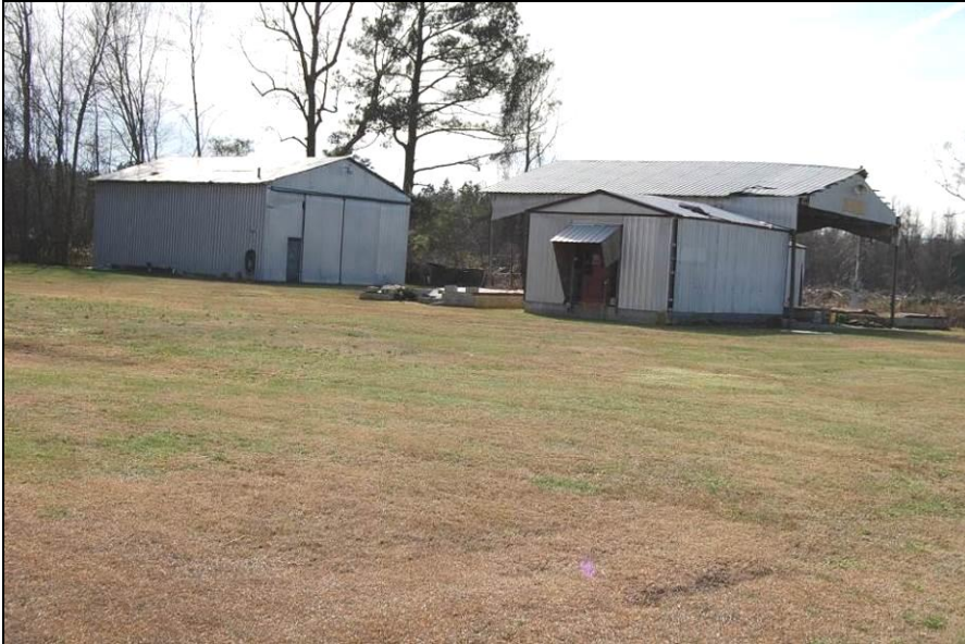
Figure 74. Willie Humphrey Farm, looking southwest at bulk barn complex at right and barn/storage building at left; note concrete pads at center and right that held additional bulk barns
