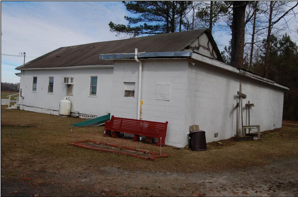
Figure 83. Foster's Chapel, west side and south rear elevations
