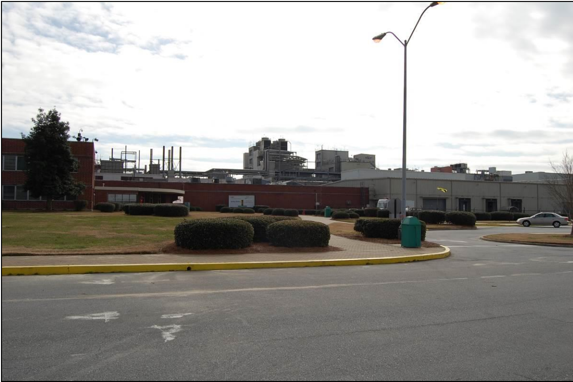
Figure 57. Looking south at facility with edge of office building at left; all buildings but for truck loading docks at right more than 50 years old
