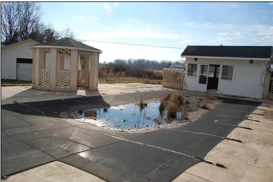
Figure 160. Looking south at pool deck with pool house at right, gazebo at left center, and storage building at far left
