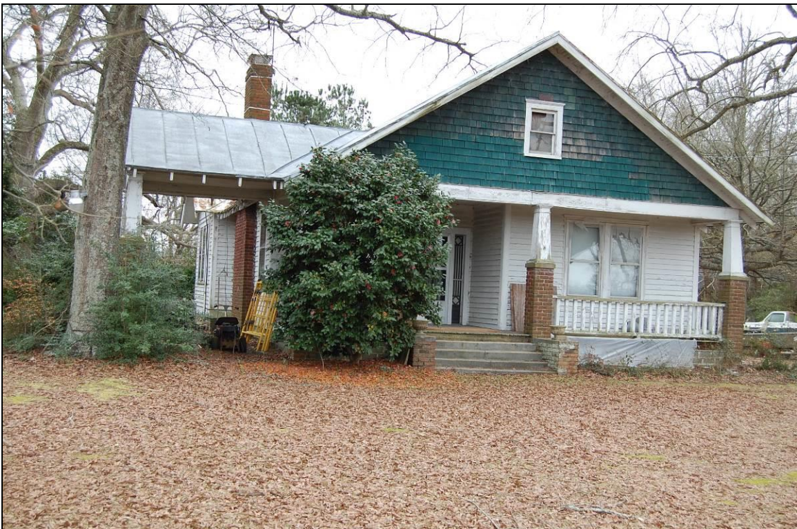
Figure 17. Southwest front and northwest side elevations of Contentnea School teacherage
