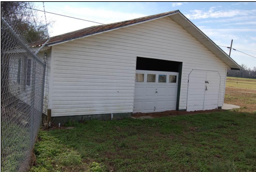
Figure 162. Looking south at storage building
