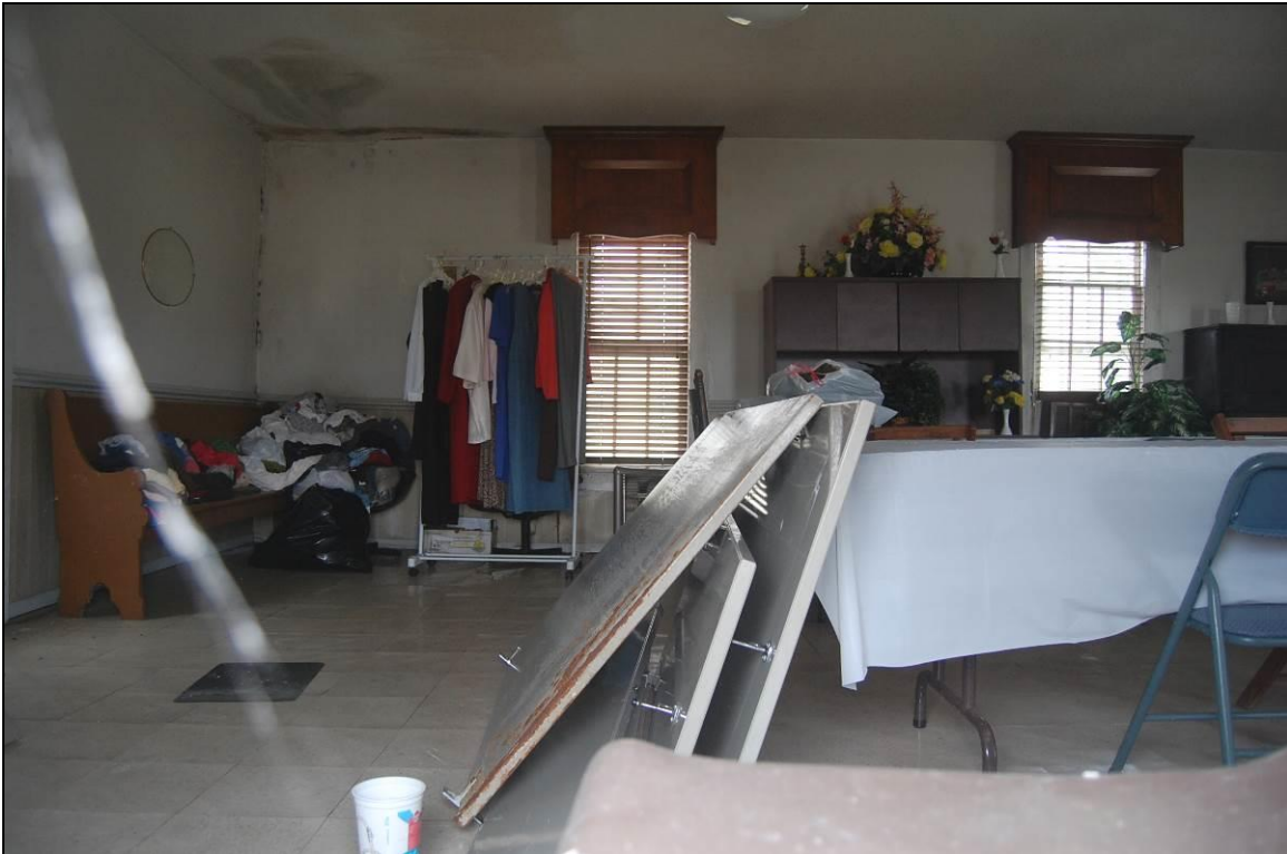
Figure 101. Interior of Jericho A.M.E. Zion Church Fellowship Hall; note modern finish and early pew at left against east wall
