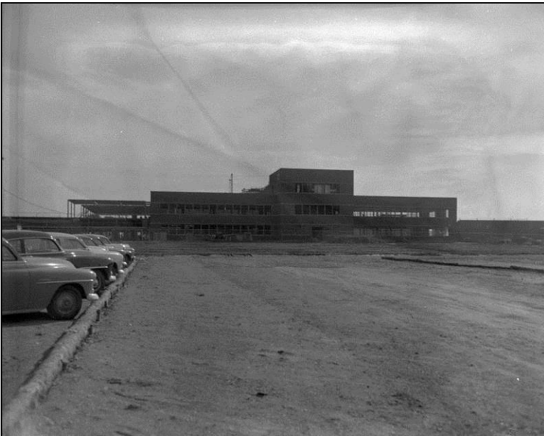
Figure 43. Plant with cladding added, 1951 (source: https://digital.lib.ecu.edu/2003 )
