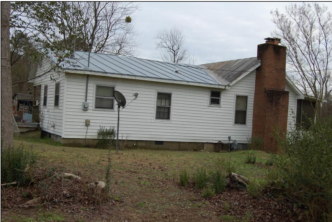
Figure 87. Eliza Dawson Farm, north rear and west side elevations of house
