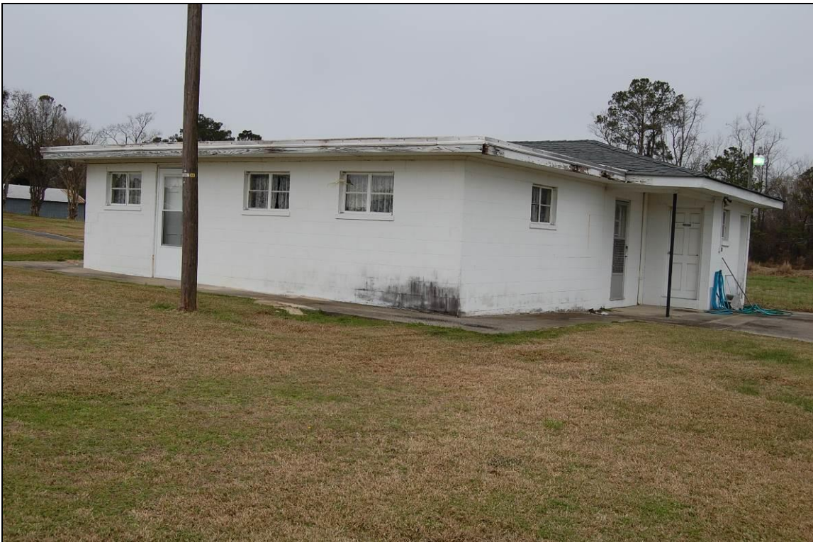
Figure 102. Looking northeast at concrete-block office
