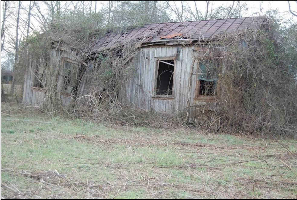
Figure 191. Graingers Railroad Section House, looking northwest
