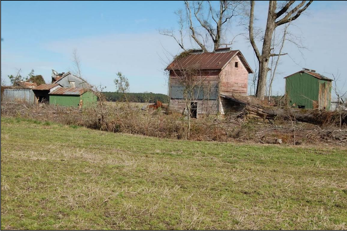
Figure 79. Willie Humphrey Farm, looking northeast at telescoping haybarns at left and frame tobacco barns at right
