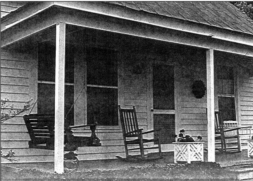
Figure 69. Willie Humphrey Farm, front elevation of farmhouse with intact weatherboards, six-over-six sash, and seam-metal roof, 1994 (photographer: Robbie Jones)
