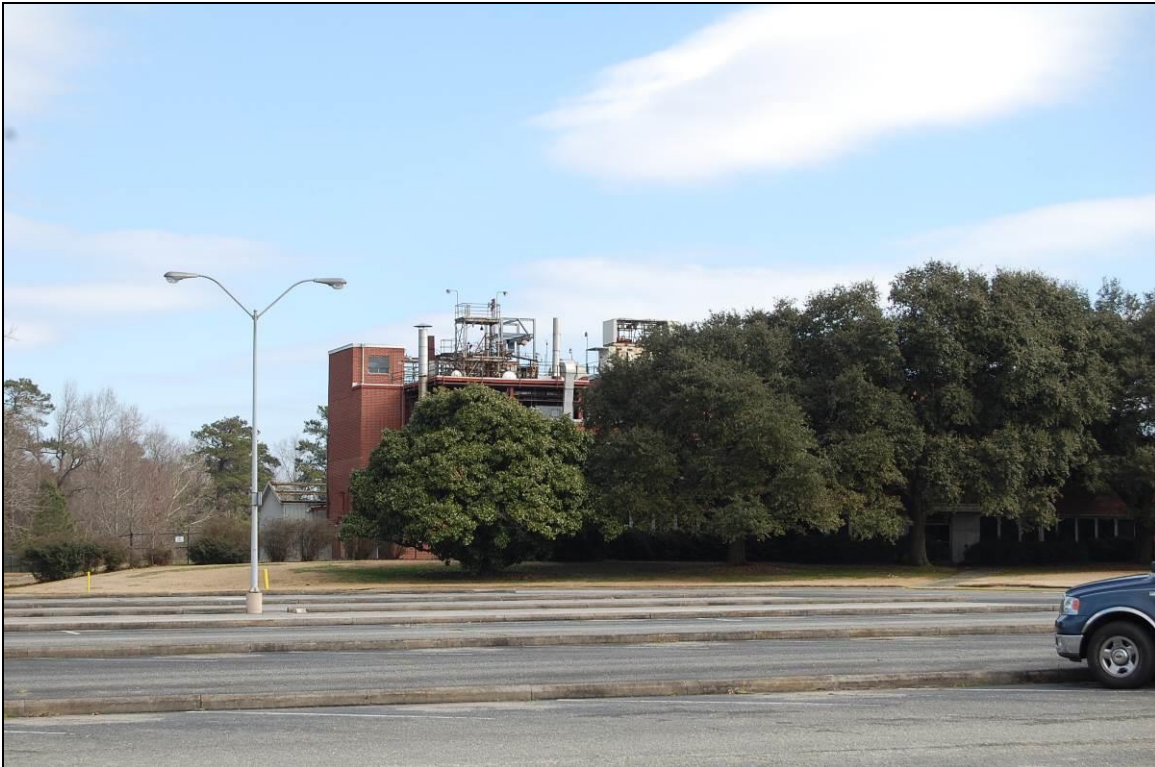
Figure 52. Looking north at laboratory building
