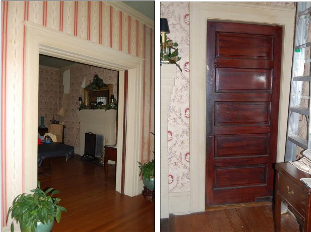
Figure 26. Charles A. Broadway House, looking from front west (right) parlor at pocket doorway into north (left) parlor; five-panel door from north parlor leading to rear rooms
