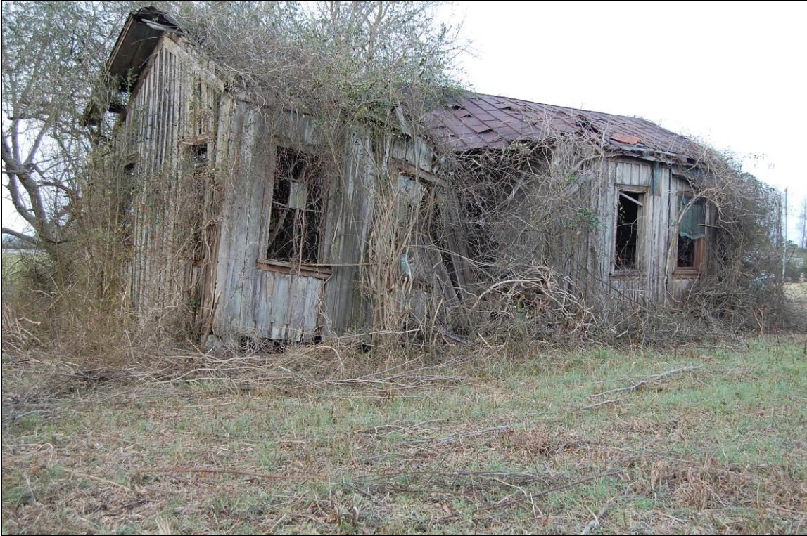
Figure 193. Graingers Railroad Section House, looking northwest
