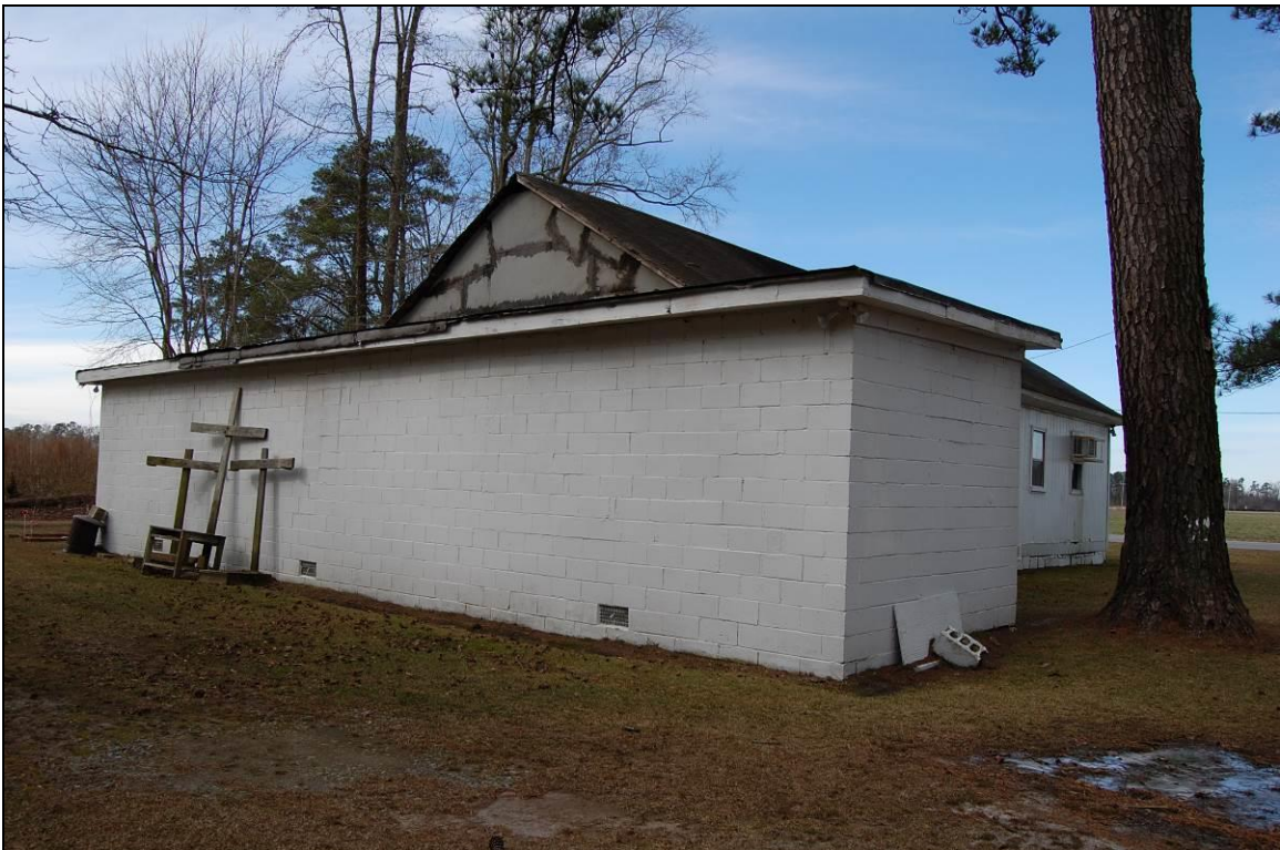
Figure 84. Foster's Chapel, south rear and east side elevations
