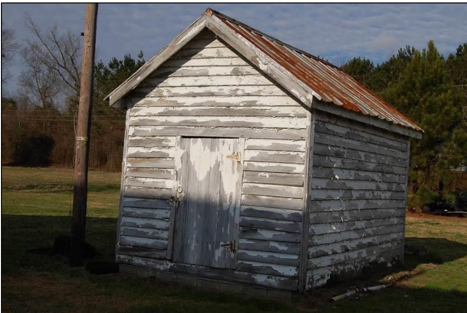
Figure 169. Looking northwest at smokehouse
