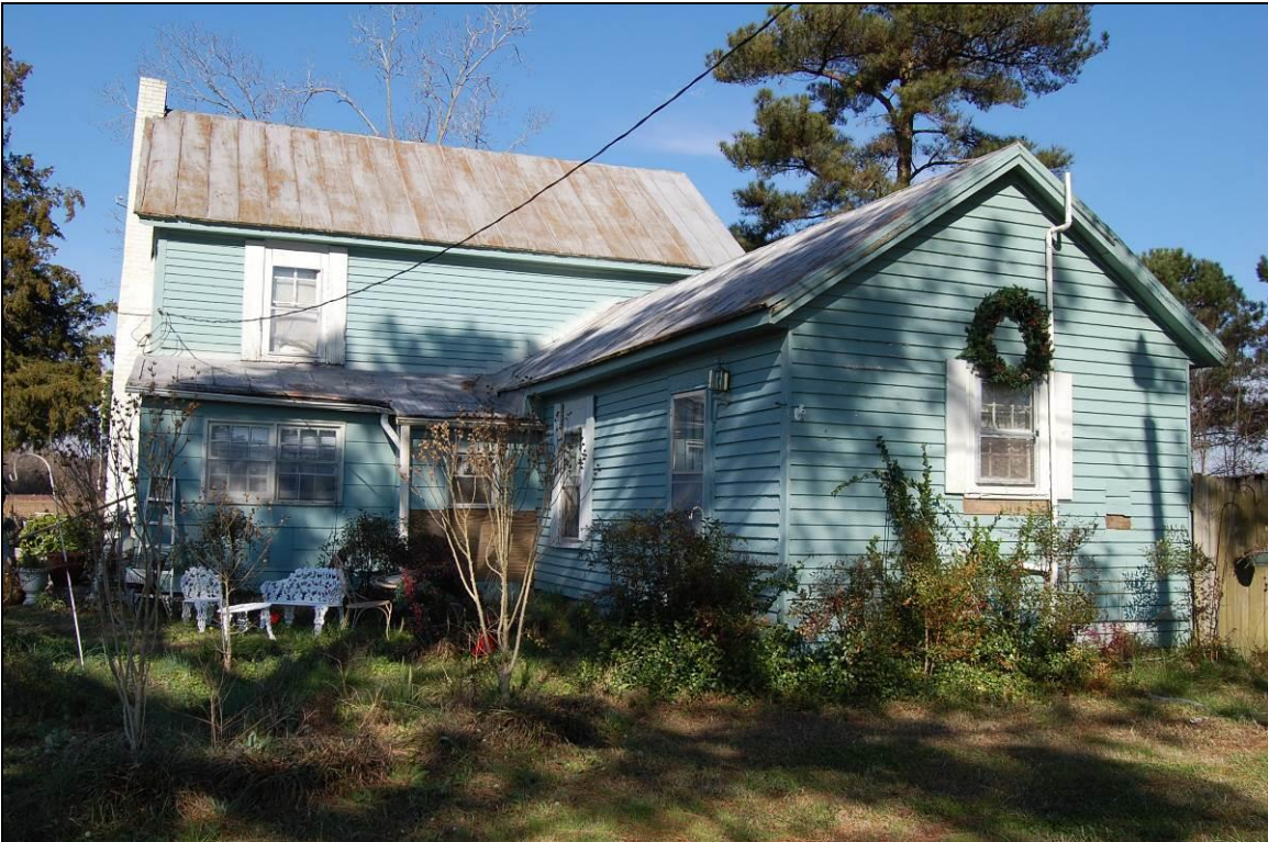
Figure 138. Southeast rear and southwest side elevations of house
