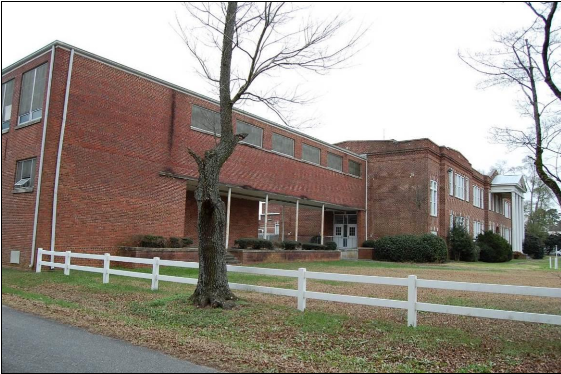
Figure 14. Southwest front and northwest side elevations of Contentnea School
