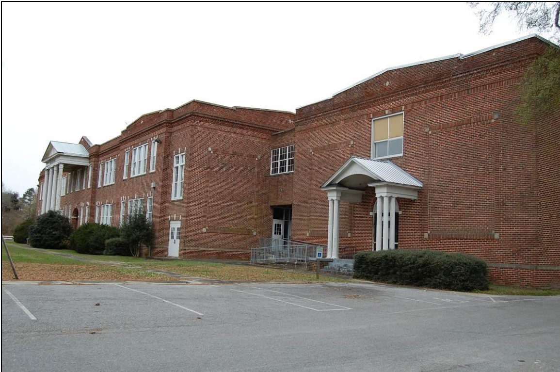
Figure 16. Southwest front and southeast side elevations of Contentnea school
