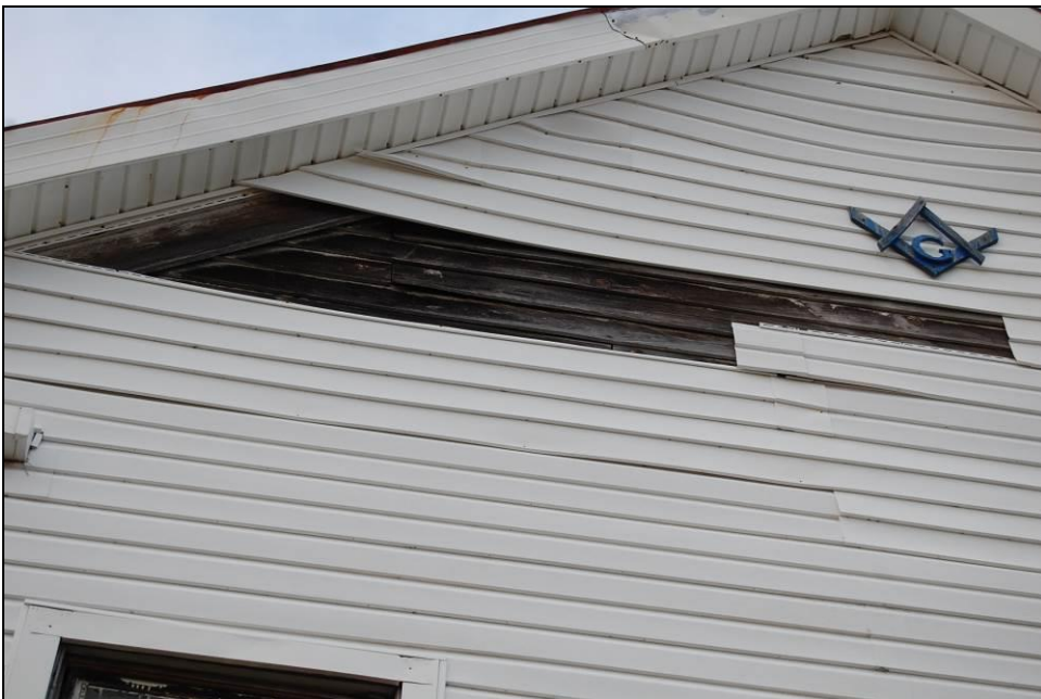
Figure 184. Southeast front elevation weatherboards and square-and-compass Masonic symbol
