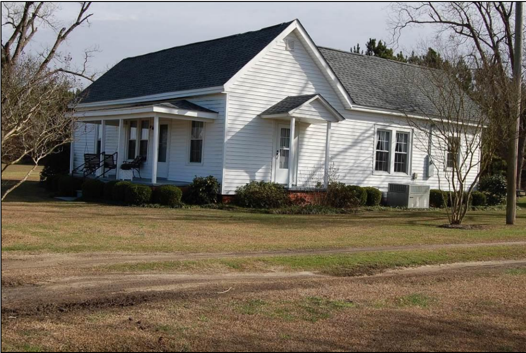
Figure 68. Willie Humphrey Farm, north front and east side elevations of farmhouse
