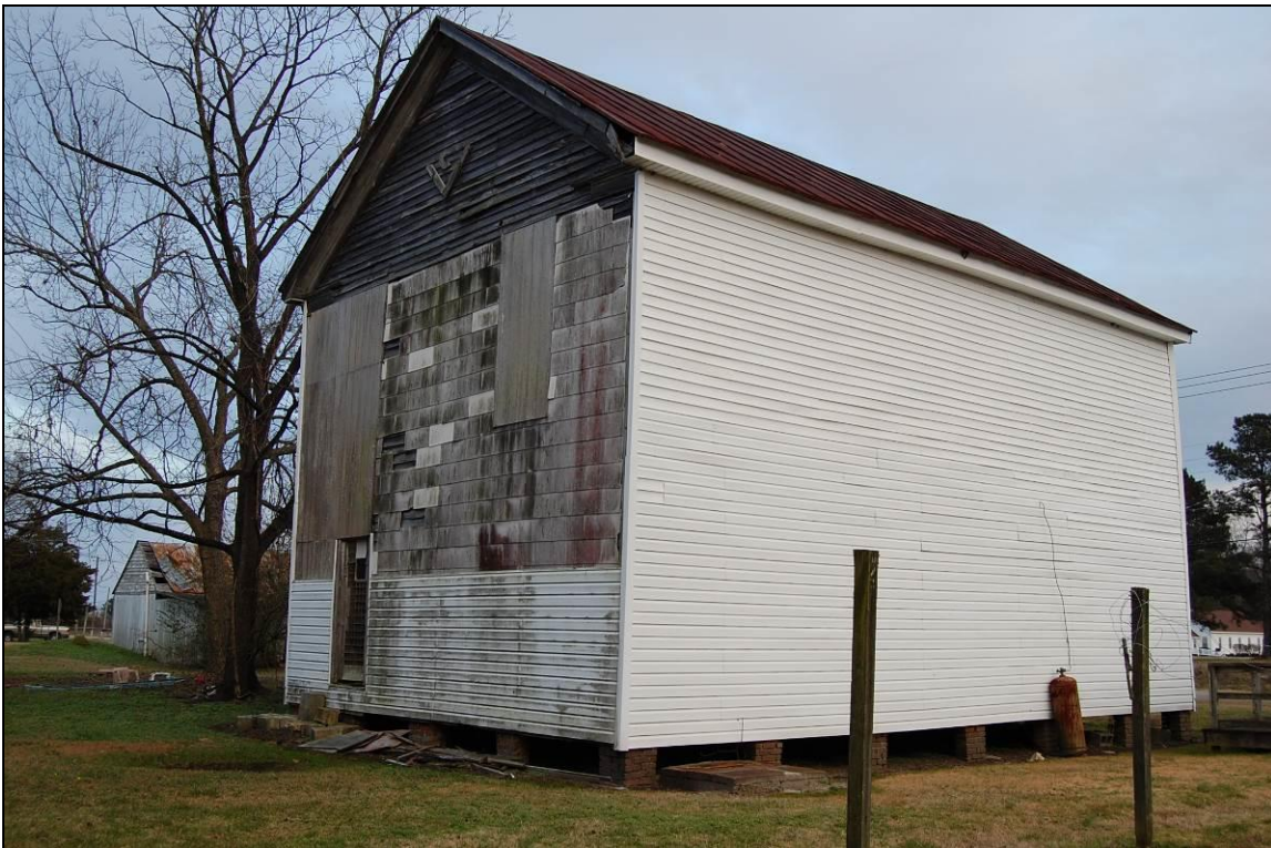
Figure 186. Southwest side and northeast rear elevations
