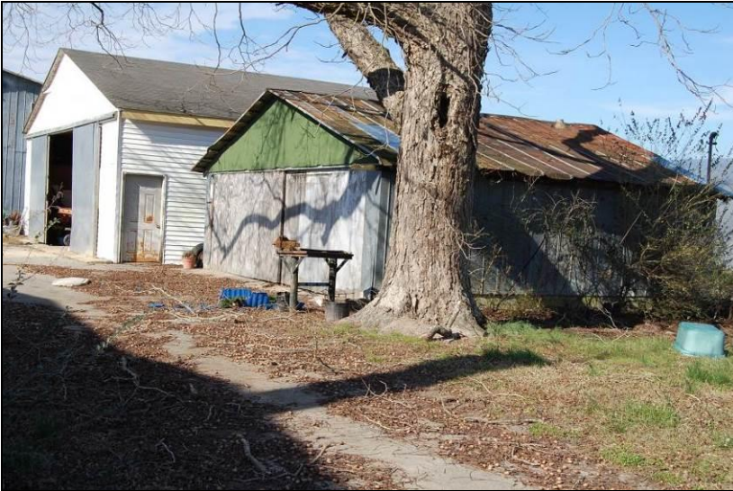
Figure 125. Looking northwest at shop at center
