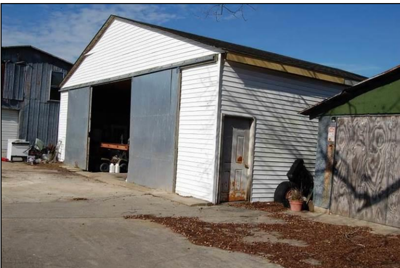
Figure 126. Looking northwest at farm equipment shed at center
