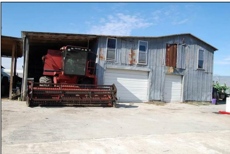
Figure 128. Looking west at packhouse/farm equipment shed
