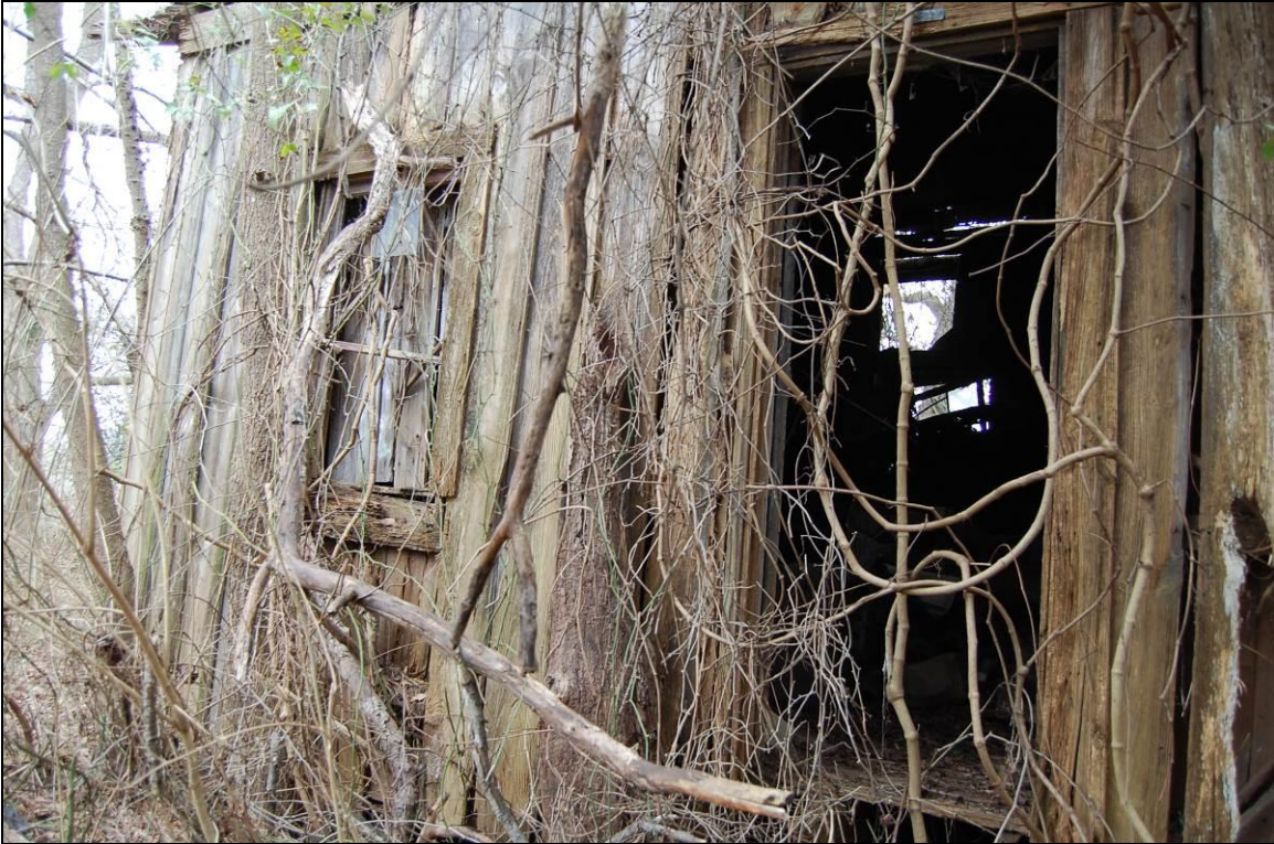
Figure 36. Two bays at left of southwest front elevation of bunkhouse
